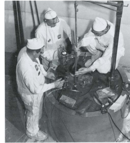
MSRE maintenance used long shafted tools
