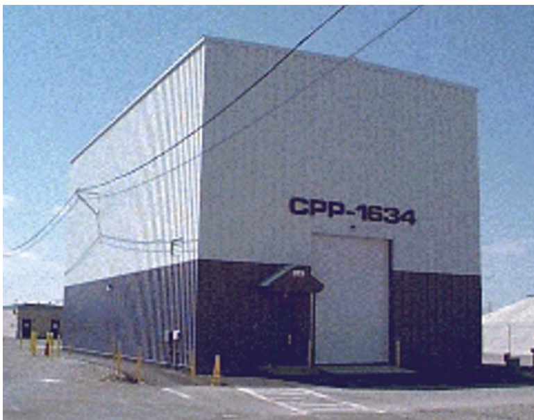
Figure 3. Building CPP-1634, located on the western edge of the Idaho Nuclear Technology and Engineering Center. The building is constructed as a large, high-bay space.
