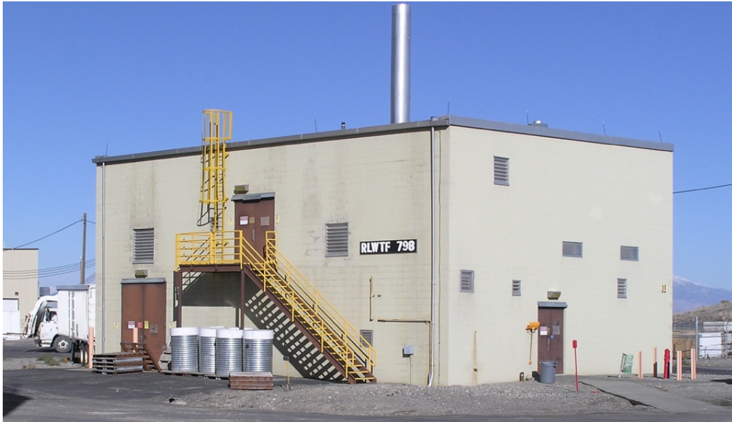
Figure 1. Building MFC-798, the Radioactive Liquid Waste Treatment Facility, a two-story, concrete-masonry block building, located in north central MFC.
