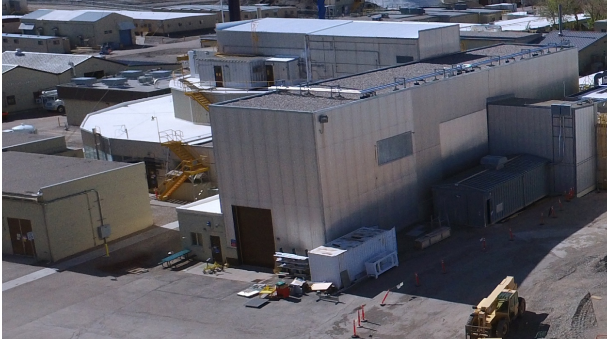
Figure 2. Photo showing the north side of MFC-765, the Fuel Conditioning Facility (FCF), located in the center of MFC. The FCF Mockup Shop area is located in north portion of the high bay shown in the foreground.
