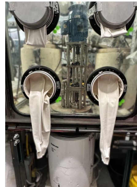
Photo of installed pump
