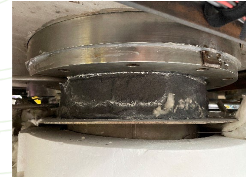
Mounted cooling coils
