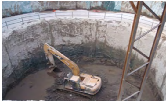
Vertical Shaft Excavation
