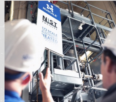
One-third scale NIST-1 Test Facility
