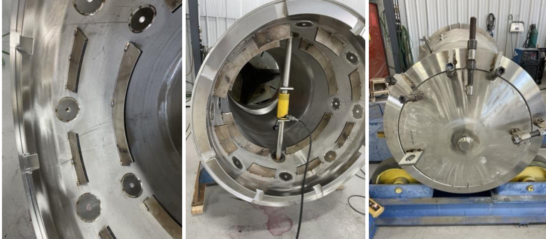
Figure 5. (Left) Strongbacks inside the guard vessel prior to welding the flanged couplings (April 2024). (Center) A hydraulic jack used in concert with strongbacks to maintain pressure on the flanged couplings during weld out , which prevented the “sinking” that had been evidenced on the sump plug to the lower cone weld (April 2024). (Right) Strongbacks and stiffeners prior to welding of the bottom cone of the guard vessel (August 2024).
