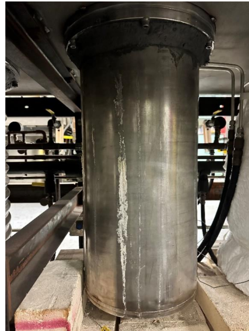
Disassembled furnace well with updated cooling system
