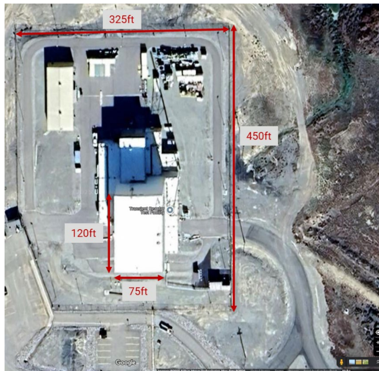
c. The TREAT facility at Idaho National Laboratory. Source: Google Maps [19].
