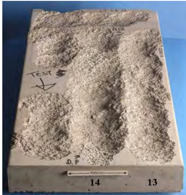
Figure C-3: Example Results of Laser Scabbling of Limestone Aggregate Concrete [1]
