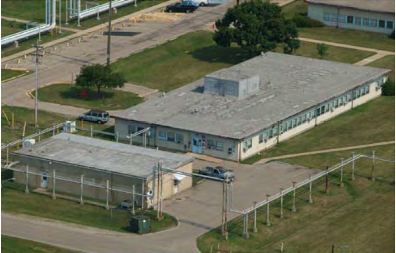
Figure 4-4: X101 Health Services Building
