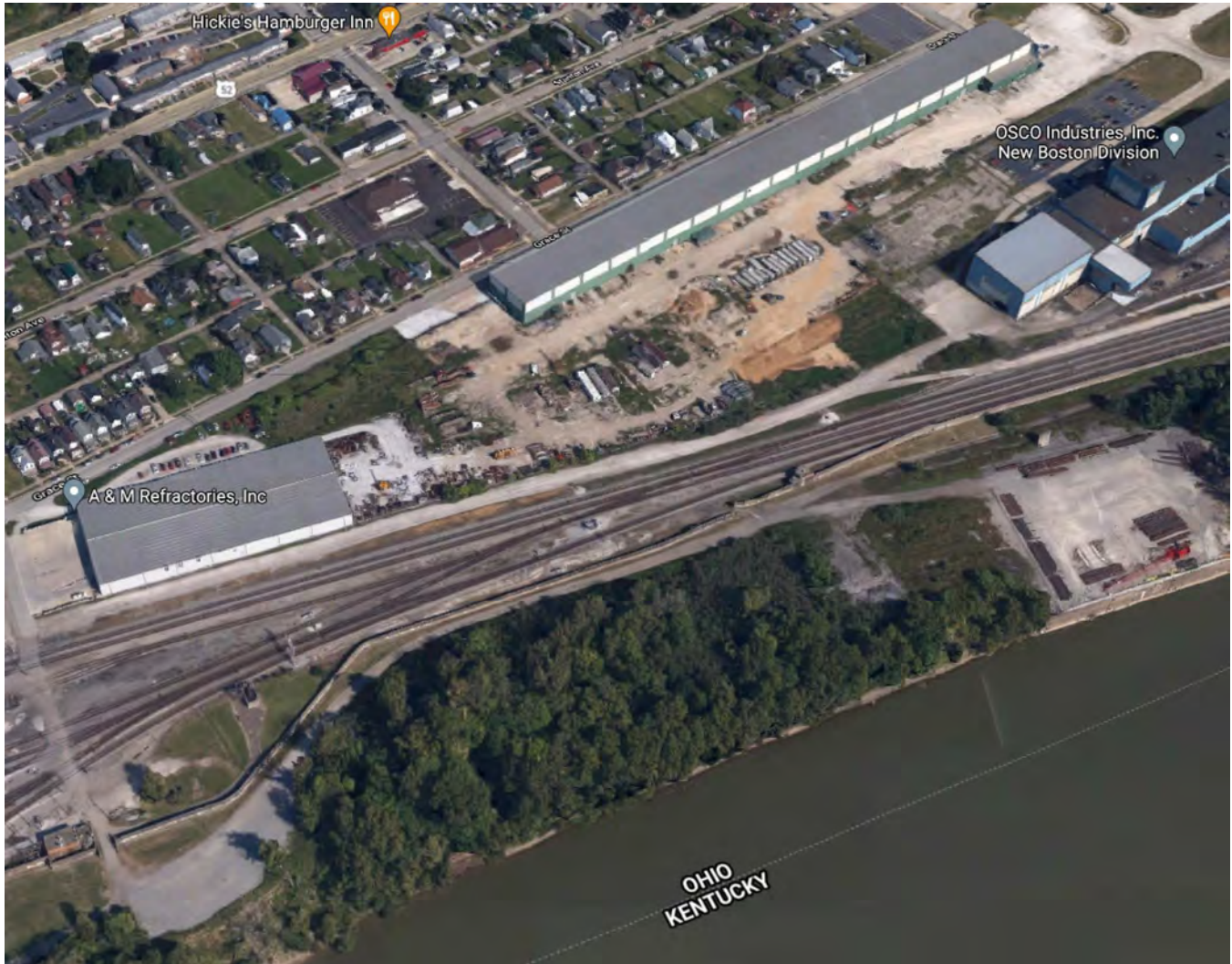
Figure 4-19: Barge access for Village of New Boston, OH
