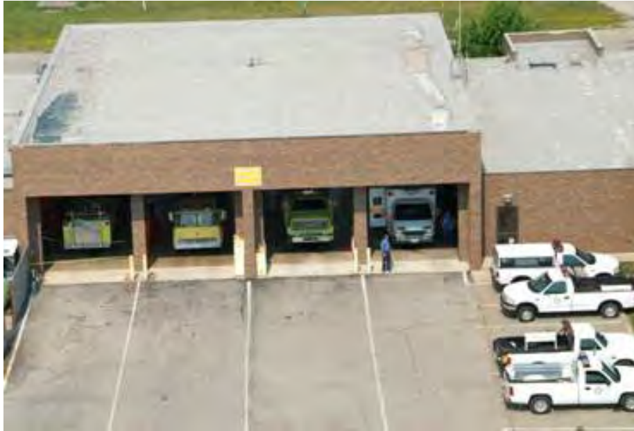
Figure 4-1: PORTS Fire Station
