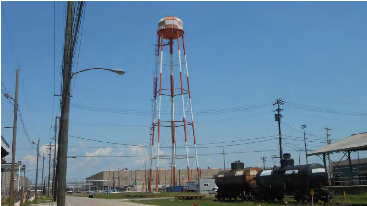
Figure 4-2: HPFW System Water Storage Tower
