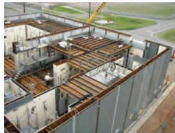
SP Reinforced Concrete
