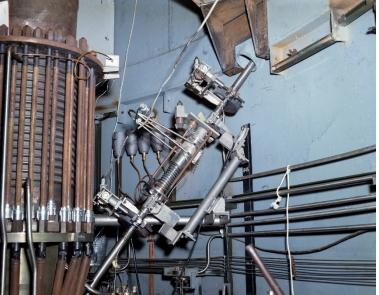
MSRE Sampler-Enricher Mechanism
