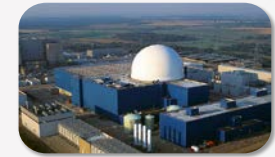
First commercial implementation (2005)
