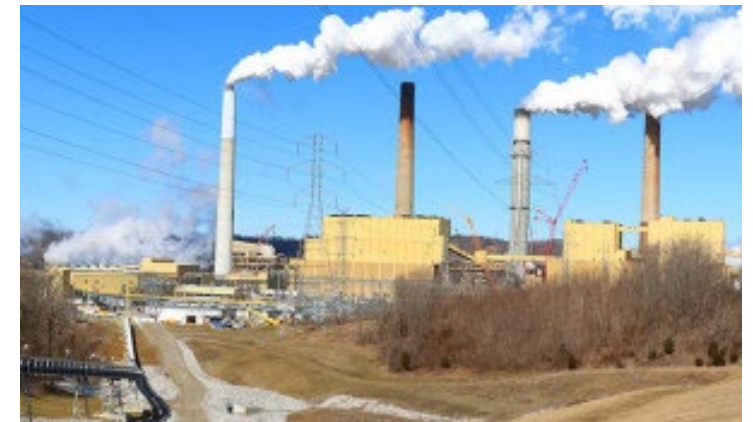
Ghent Generating Station Owned/Operated by Louisville Gas and Electric Company and Kentucky Utilities Company Located in Carroll County, KY
