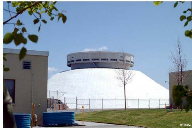
ZPPR Reactor Cell
